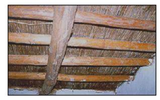
Figure 1.11 A timber floor structure in Nepal (source: WHE Report 74)
