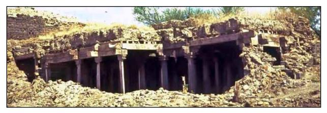
Figure 2.19 Wall collapse in the 1993 Maharashtra, India, earthquake: a stone masonry building with a timber roof and a heavy mud overlay (photo: S. Brzev)
