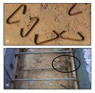
Figure 3.18 Inadequate bending of reinforcement in RC bands: a) links, and b) ties (photos: Smart Shelter Foundation)
