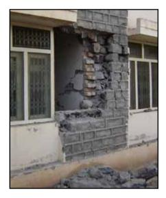
Figure 2.38 Vertical cracking at a wall intersection in the 2005 Kashmir, Pakistan, earthquake due to absence of connection between the intersecting walls, a stone masonry and a brick-masonry wall (source: Bothara and Hiçyılmaz 2008)
