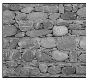
Figure 1.27 Stone masonry wall built using round river stone boulders with shaped exterior surfaces near Balakot, Pakistan (photo: T. Schacher)
