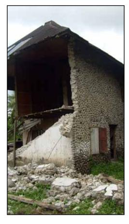
**Figure 2.30** Out-of-plane collapse of stone masonry walls in buildings with flexible roofs and inadequate wall-to-roof connections: a) the 2005 Kashmir, Pakistan, earthquake (photo: M. Tomazevic); b) the 2003 Boumerdes, Algeria, earthquake (photo: M. Farsi)
