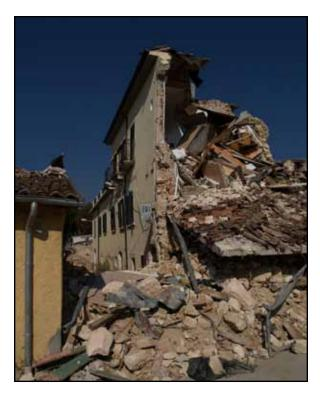
Figure 2.1 Extensive damage to stone masonry buildings in the 2009 L'Aquila, Italy, earthquake (photo: T. Schacher)
