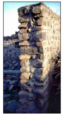
Figure 3.27 Examples of stone masonry in cement mortar with a wall thickness limited to 450 mm (note through-stones) (photos: S. Brzev)
