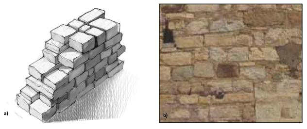
Figure 1.31 Dressed stone masonry: a) an isometric view of a typical wall, and b) an exterior of a wall in Umbria, Italy (source: Maffei et al. 2006)
