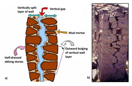
Figure 2.20 Delamination of stone masonry walls: a) delamination in progress (source: Murty 2005), and b) delamination of wall wythes due to the 1993 Maharashtra, India, earthquake (photo: S. Brzev)
