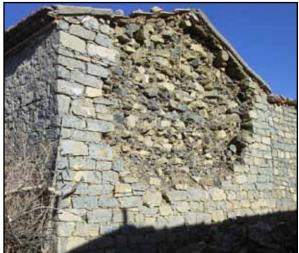
Figure 2.22 Delamination of a stone masonry wall in the 2000 Beni-Ouartilane, Algeria, earthquake (photo: M. Farsi)
