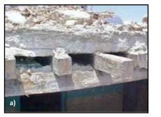
Figure 2.14 Roof deficiencies in the area affected by the 2001 Bhuj, India, earthquake: a) discontinuous rafters over interior walls, and b) inadequate wallto-floor connections caused the severe building damage (photos: C.V.R. Murty)
