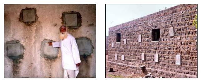
Figure 4.20: Examples of completed through-stone retrofit projects in Maharashtra, India (photos: S. Brzev)
