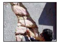
Figure 2.37 A stone masonry wall with thick mud mortar (thickness on the order of 80 mm) in the area affected by the 2001 Bhuj, India, earthquake (photo: J. Arlekar)
