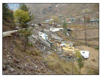
Figure 3.1 A collapsed building on a steep slope after the 2005 Kashmir earthquake, Pakistan (source: Bothara and Hiçyılmaz 2008)
