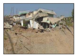
Figure 3.3 A building damaged by a landslide in the 2005 Kashmir, Pakistan, earthquake (source: Bothara and Hiçyılmaz 2008)
