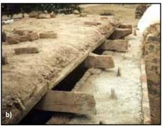
**Figure 4.6** An example of a field application of an RC band in an existing stone masonry building in Maharashtra, India: a) RC band installation completed (note brick edging at the band level and a newly constructed portion of the wall above the band), and b) RC band at the roof level underneath the timber beams (note that the roof is supported by an interior timber frame) (photos: S. Brzev)
