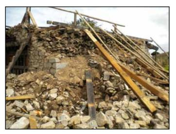
Figure 2.4 Collapsed stone masonry buildings, 2009 Bhutan earthquake (photo: K. Vatsa)
