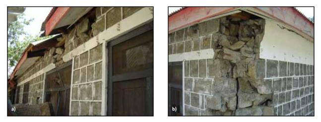
Figure 2.11 A stone masonry building with an RC lintel band that survived the 2005 Kashmir earthquake in Pakistan: a) the building suffered only moderate damage in the top portion, and b) separation at the wall intersection took place in spite of the band (note inadequate anchorage of the band reinforcement) (photos: Builders Without Borders)
