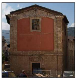
Figure 2.16 A building with roof-to-wall anchors survived the 2009 L'Aquila, Italy, earthquake (photos: T. Schacher)
