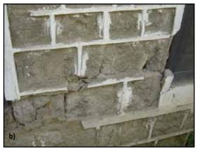
Figure 2.34 Shear failure in stone masonry walls: a) shear cracks initiated at the corners of openings in the 2005 Kashmir, Pakistan, earthquake (Photo: Bothara and Hiçyılmaz, 2008), and b) shear cracking in a stone masonry pier damaged by the same earthquake (photo: Builders Without Borders)
