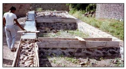
Figure 3.39 Construction of an RC plinth band using large stone rubble (also known as "stonecrete") (photo: S. Brzev)
