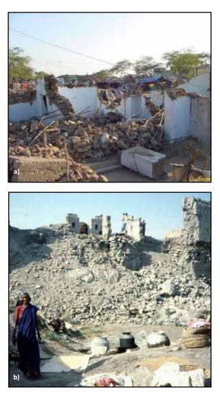
**Figure 2.2** Extensive damage to stone masonry buildings in Indian earthquakes: a) the 2001 Bhuj, Gujarat, earthquake (photo: C.V.R. Murty), and b) the 1993 Maharashtra earthquake (photo: S. Brzev)
