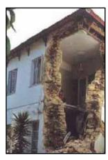
Figure 2.7 Vertical crack in a stone masonry wall due to the 1993 Maharashtra, India, earthquake (photo: S. Brzev)
