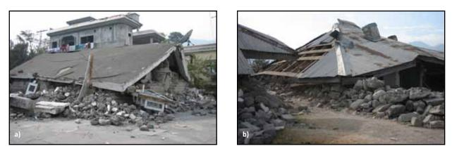
Figure 2.18 Collapse of roof structures due to the loss of gravity load-bearing capacity of stone walls in the 2005 Kashmir, Pakistan, earthquake: a) reinforced concrete roof, and b) timber and steel roof (photos: M. Tomazevic)
