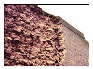
Figure 2.23 Delamination was a common damage pattern observed in the 1993 Maharashtra, India, earthquake (photos: S. Brzev)
