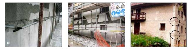
Figure 4.4 A field application of ties in Slovenia: a) and b) installation of steel ties after the 1998 Bovec, Slovenia, earthquake (note that anchorage end-plates are yet to be attached), and c) an example of a retrofitted building (photos: M. Lutman)
