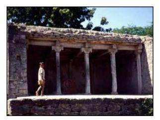
**Figure 1.12** A timber roof structure with mud overlay in Maharashtra, India (photo: S. Brzev)
