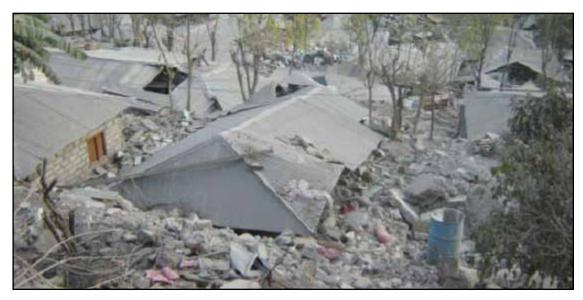
Figure 2.17 Collapse of stone masonry buildings with hipped roofs in the 2005 Kashmir, Pakistan, earthquake (source: Bothara and Hiçyılmaz 2008)
