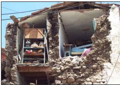
Adequate connections between cross walls and long walls are critical for preventing out-ofplane wall collapse.
