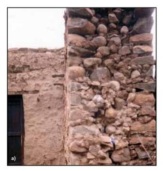
Figure 1.22 Typical uncoursed random rubble stone walls: a) an uncoursed random rubble stone wall in Maharashtra, India, showing exterior wythes and stone rubble in mud mortar in between (photo: S. Brzev) and b) plan view of a stone wall under construction in Nepal (note stone rubble
