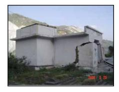
**Figure 2.39** Soil spreading in the 2005 Kashmir, Pakistan, earthquake - note wide cracks in the walls (source: Bothara and Hiçyılmaz 2008)
