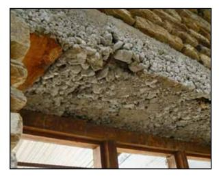
Figure 3.20 Poor concrete construction quality in an RC lintel band (photo: Smart Shelter Foundation)
