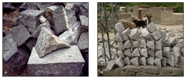
Figure 1.21 Semi-dressed stones ready for wall construction: a) wedged stones in Maharashtra, India (photo: S. Brzev), and b) shaped stones in Pakistan (photo: T. Schacher)
